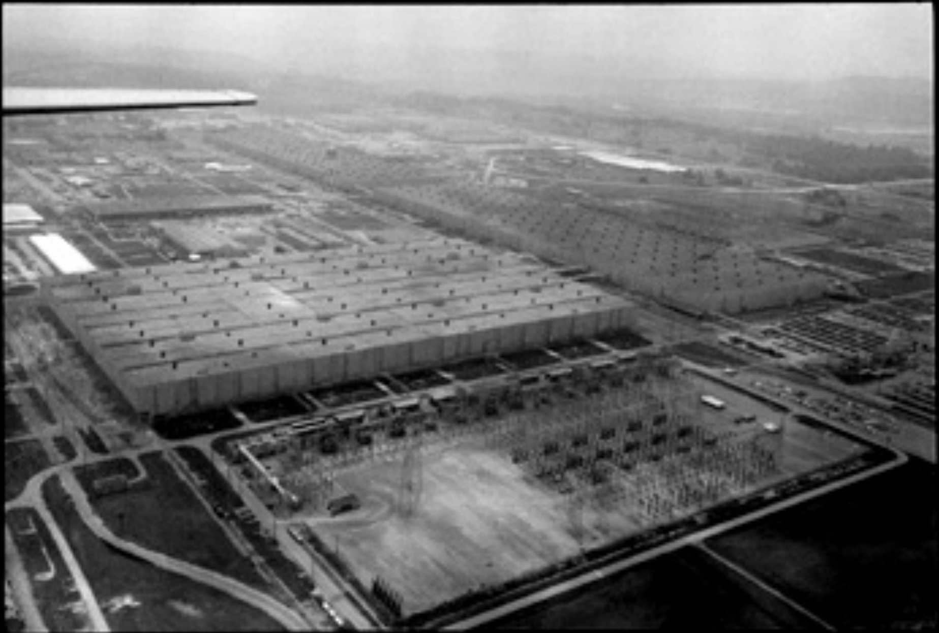
Uranium enrichment plant – increases U-235 content
