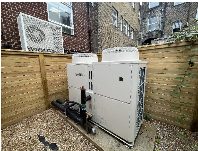
Figure 1: Air Source Heat Pumps at Upper Norwood Library.
